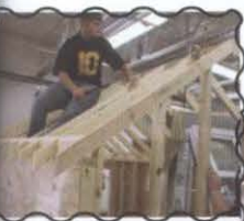
Nick works on the shed. Literally.
